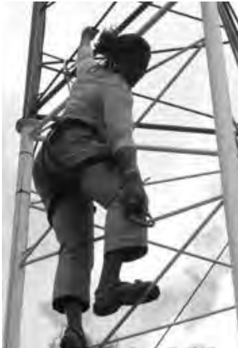
Figure 11.3: Omelayo Samuel, one of the staff of Zittnet, does not fear the height of the 45m tall tower as she is aligning the antennas hosted in the top of the tower.
